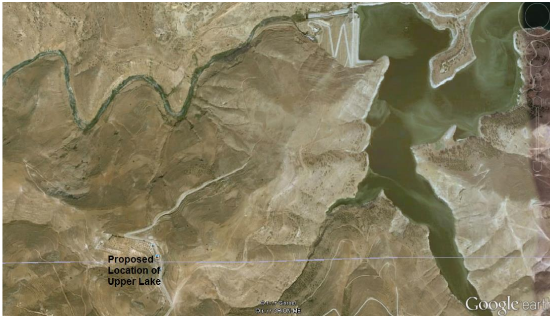
Figure 2 King Talal dam showing the lower lake and the location of the upper lake
