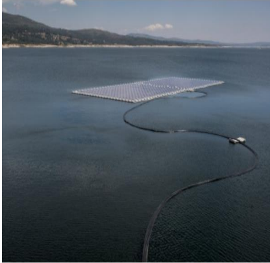
Figure (1) The first solar-hydro integrated system in Portugal.
